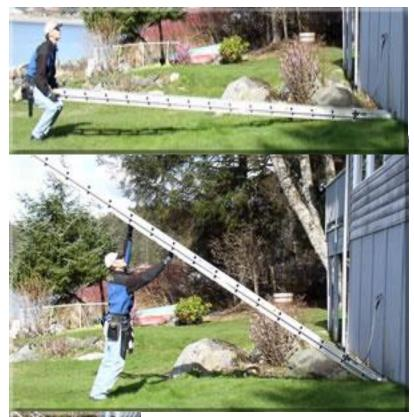
**Second** - lift ladder's top while pushing forward to maintain pressure against building's wall. \*Don't perform ladder work if you are not mentally or physically capable of safely accomplishing the work. \*Lift with your legs, not your back.
