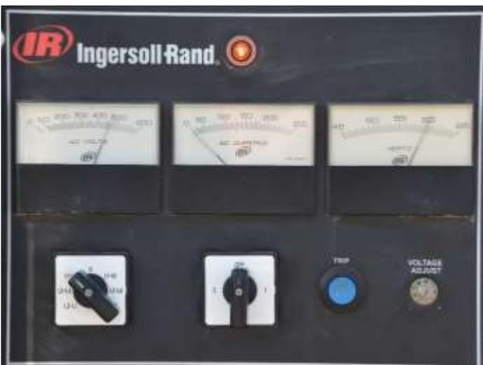
The panel selector switches show how much Voltage and Amperage is being generated between each lug. **Note:** The amp meter will only register when there is a load hooked to the generator.
